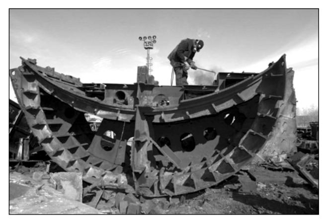
As part of the Nunn-Lugar/Cooperative Threat Reduction Program; A Russian shipyard worker uses a cutting torch to breakdown a large bulge section of a Russian Oscar Class submarine at the shipyard in Severodvinsk.
